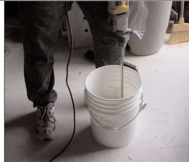
Use Proper Mixing Equipment
